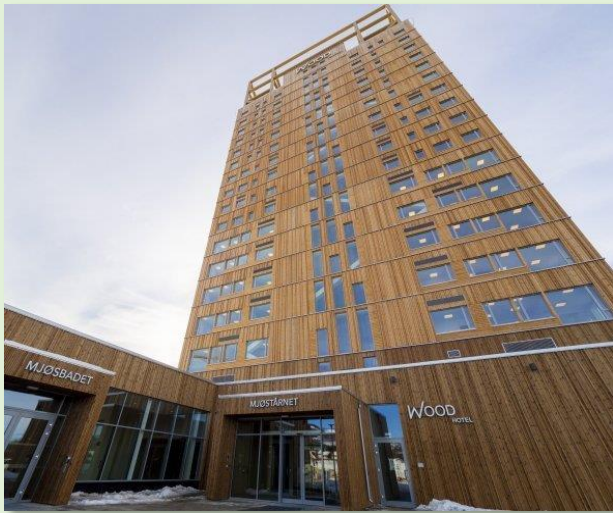
The 18-story building north of Oslo in Mjøstårnet
