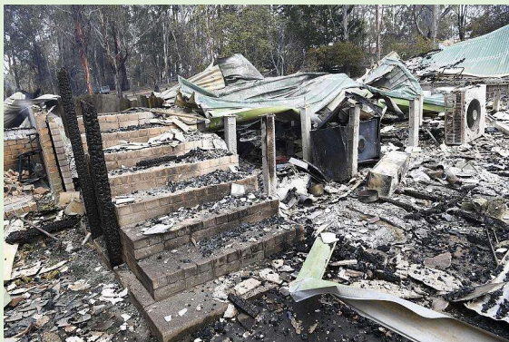
An example of the resulting devastation and destruction.
